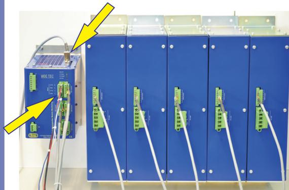
Connection of the RS485 bus and of the message contact from the UCC-TEC to the process control system
